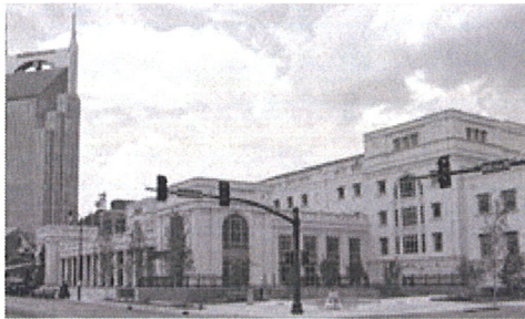
The Nashville Schermerhorn Symphony Center is shown here nearing completion. Photo by Anita Blake.
