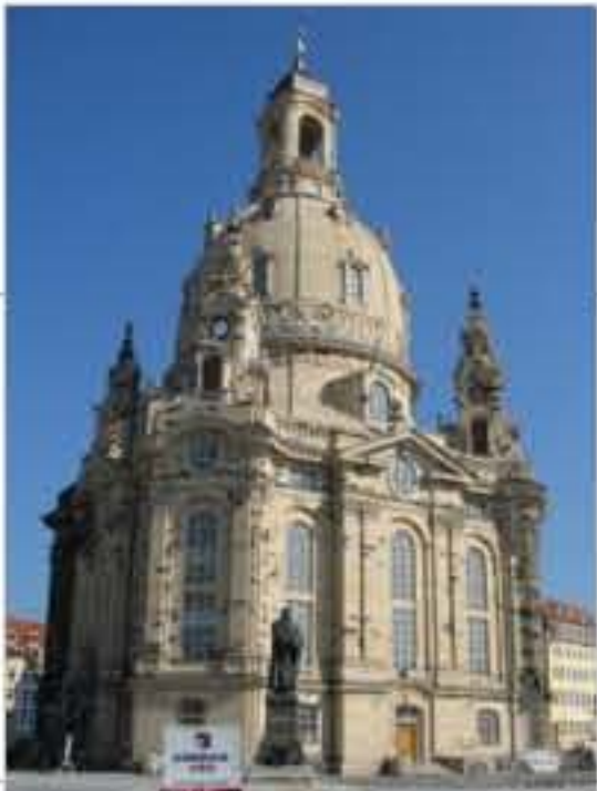
The Dresden Frauenkirche, in Dresden Germany, was rebuilt after the British bombing in the Pan-Global War destroyed it. Its meticulous rebuilding, true to its original design, lasted from 1994 to 2004 (with the interior completed in 2005).
